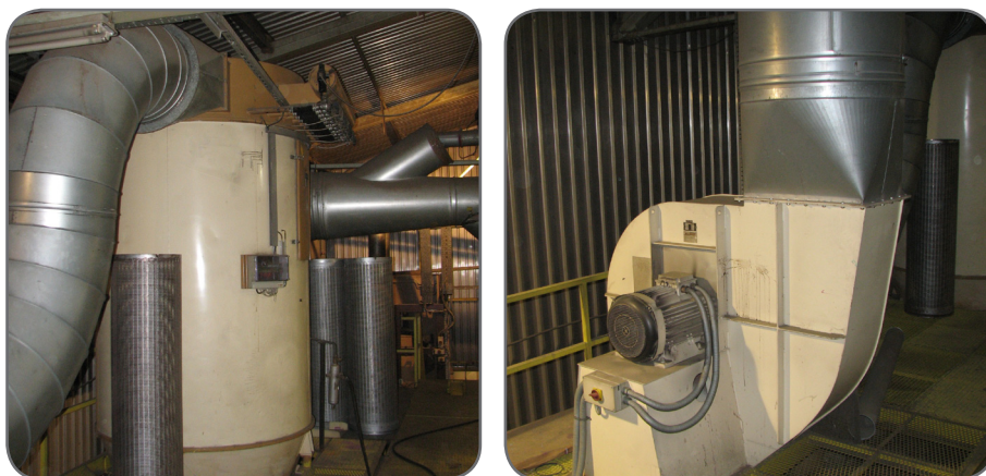
Slika 18. Filter ciklon Figure 18. Cyclofan (Prole, 2009)
